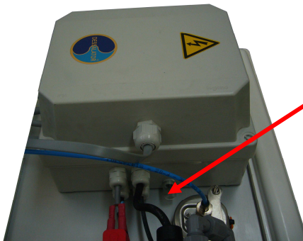
Pump cable case 220V
