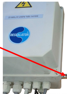
Pump cable case 380V
